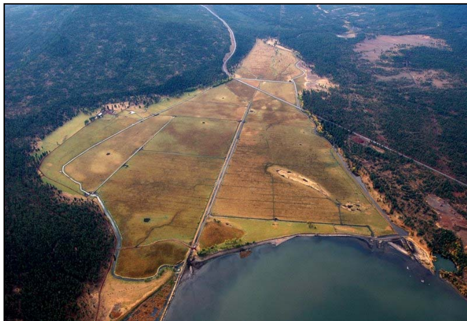
Figure 3-4. Aerial photo of Ditched portion of Denney Creek (DEA 2009).
